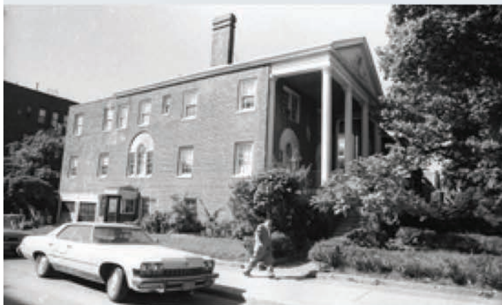
THE MECHNEH YISROEL HOUSE, CORNER OF PRESIDENT STREET AND KINGSTON AVENUE IN CROWN HEIGHTS.
